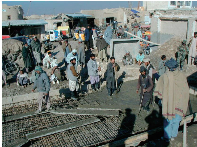
Road construction work in Kandahar Photo courtesy of Shozo Kawasaki
