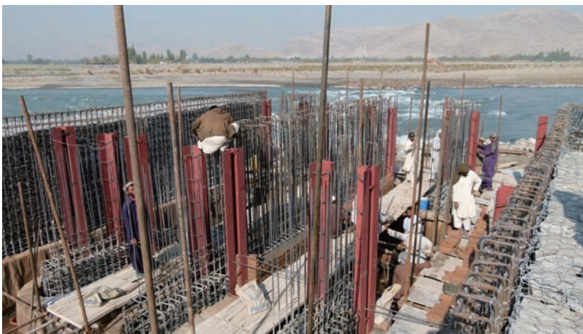
Farmers working on inlet weir construction Photo: Peace (Japan) Medical Services
