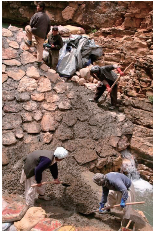
Local villagers working on construction
