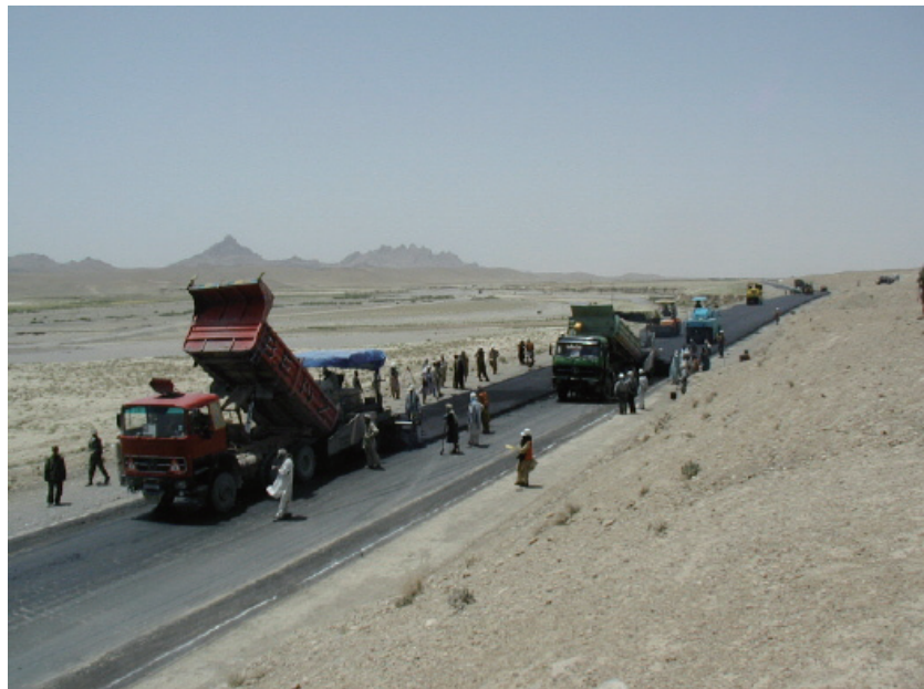
Construction work of the KK Road Photo: Toshiyuki Nose
