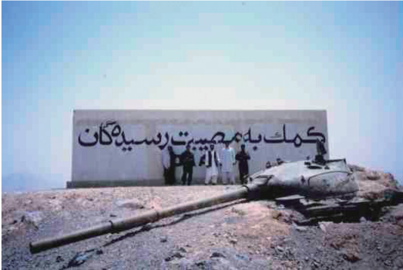
Concrete water tank built in 1973 by Japanese assistance in Kandahar (photo taken in May 2005) Photo: Hisao Ushiki
