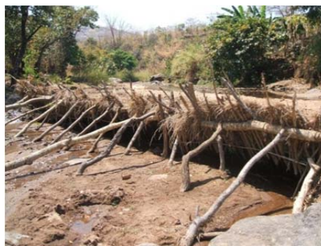
An example of temporary irrigation (an intake structure made of wooden poles and grass)
